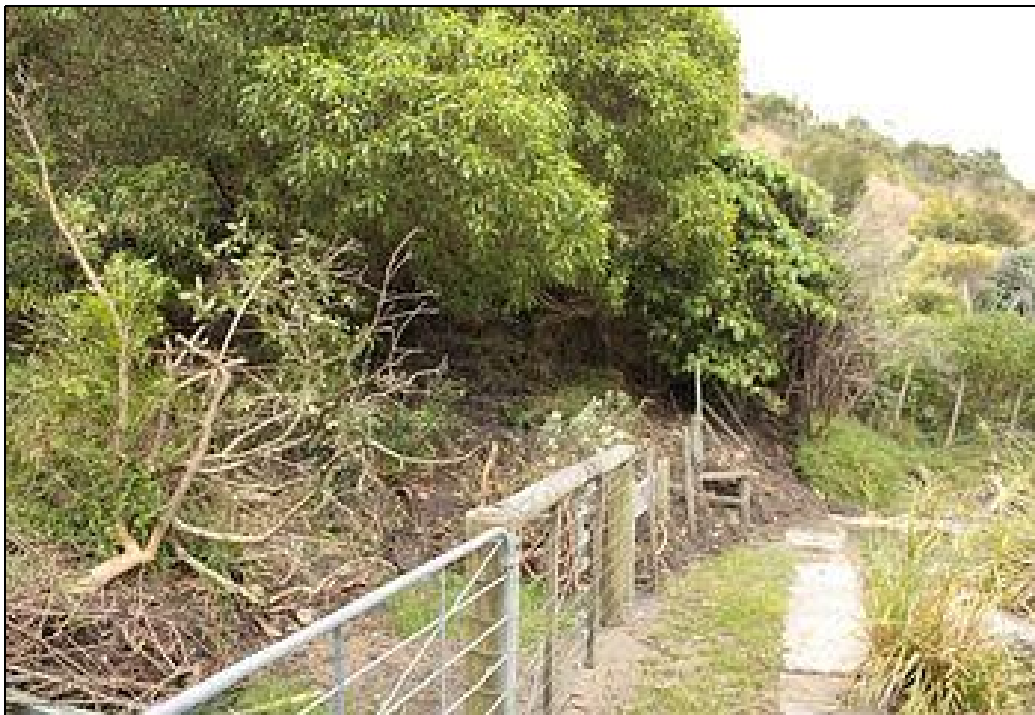
The track junction after the slip
