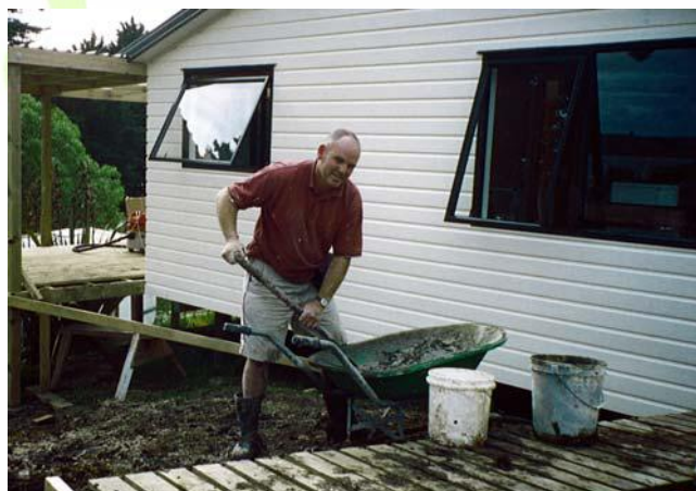
Iain Reid mixing cement for deck supports
