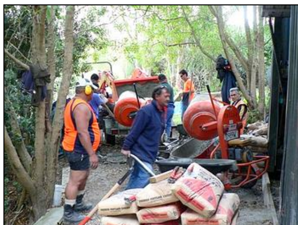
Preparation and action on the day concreting the shed floor
