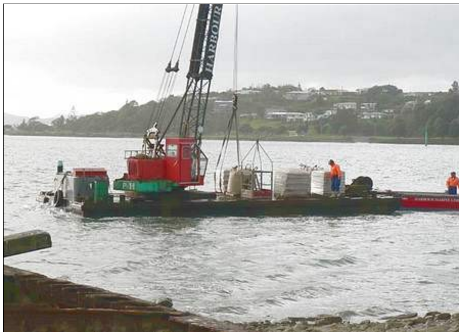
Hylton delivering the cement.
